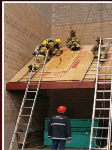
FAR LEFT: The five-story structure contains a building within a building to provide for year-round training even in inclement weather.
